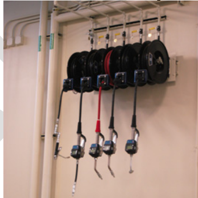
Figure 4-51 Fluids Distribution System
