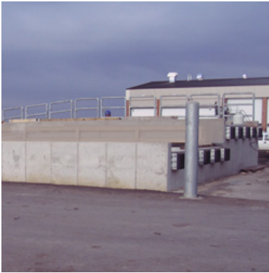
Figure 3-6 Bi-Level Loading Ramp
