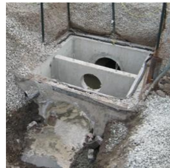
Figure 3-1 Outlet Control Structure, ARC, Wilmington,
