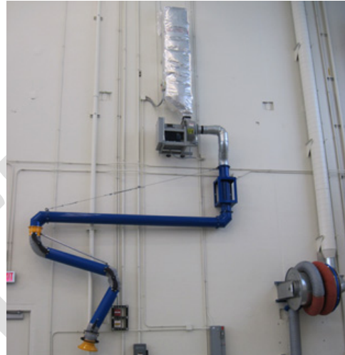
Figure 4-49 Exhaust Arm for Welding
