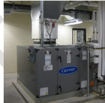
Figure 3-11 Air Handling Unit
