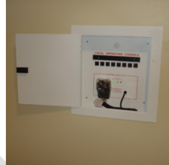
Figure 2-7 Local Operating Console (LOC) for Mass Notification
